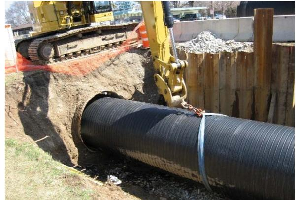
Different ways to inserting Weholite liner into the host pipe.
