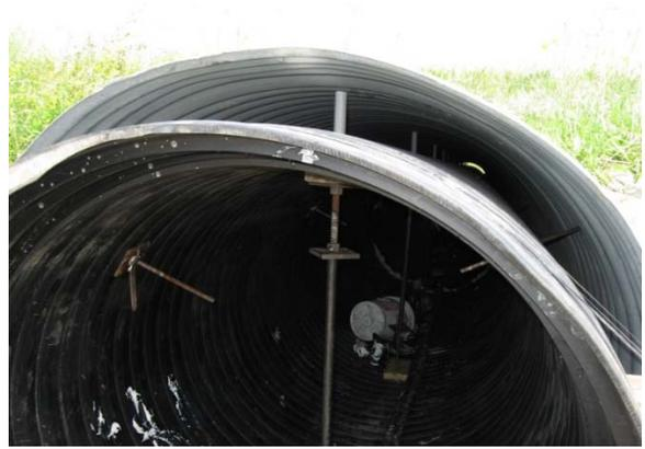
Using jacks to hold the pipe down.
