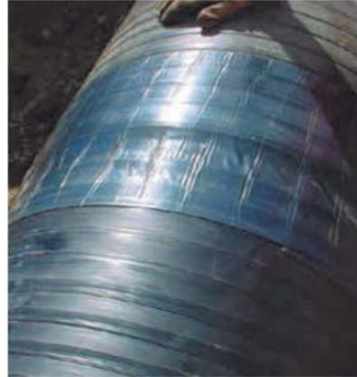
Method 2: Wehoseal joint wrap may be used to seal threaded connection. Installation is performed in the field using a propane torch and a hand roller.
