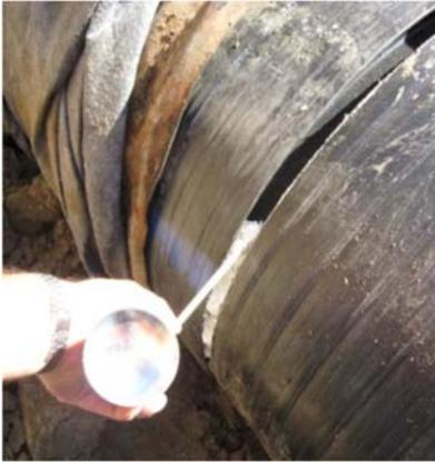
Method 1: Using Polyurethane spray foam, spray foam in joint around entire circumference of the pipe. Wipe off excess foam if necessary.
