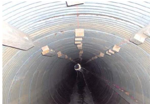
Where the blocking comes into contact with the pipe, the surface area of the blocking must be large enough to distribute the buoyancy force without distorting the pipe. When minor bends need to be navigated without the use of elbows, a side rail should be used to prevent the leading edge of the relined pipe from getting hung up on the host pipe while advancing the relined pipe.
