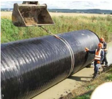
Step 3: Use nylon slings with lever or excavator arm to rotate the pipe.
