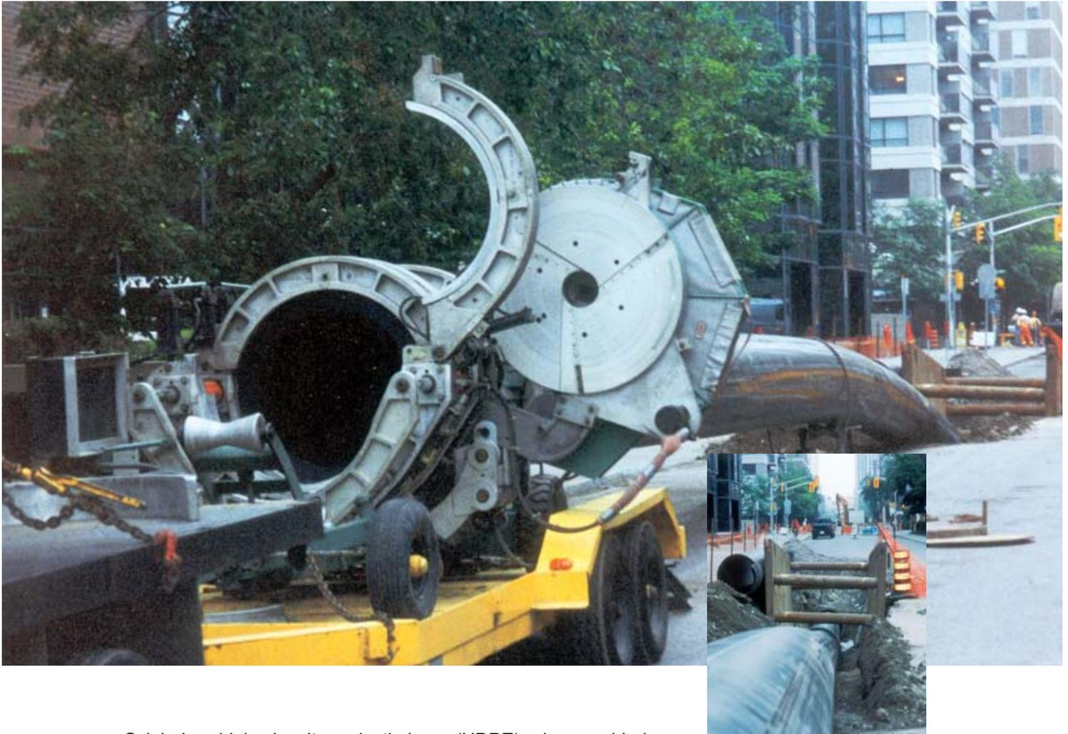
Sclairpipe high density polyethylene (HDPE) pipe enabled the Region of Ottawa – Carleton to save time and money during the restoration of a deteriorating 915 mm (36”) diameter cast iron watermain. During the busy summer months, the 82-year-old cast iron watermain under Gloucester Street (one of the busiest streets in downtown Ottawa) was sliplined with Sclairpipe, instead of using traditional open-cut construction.
