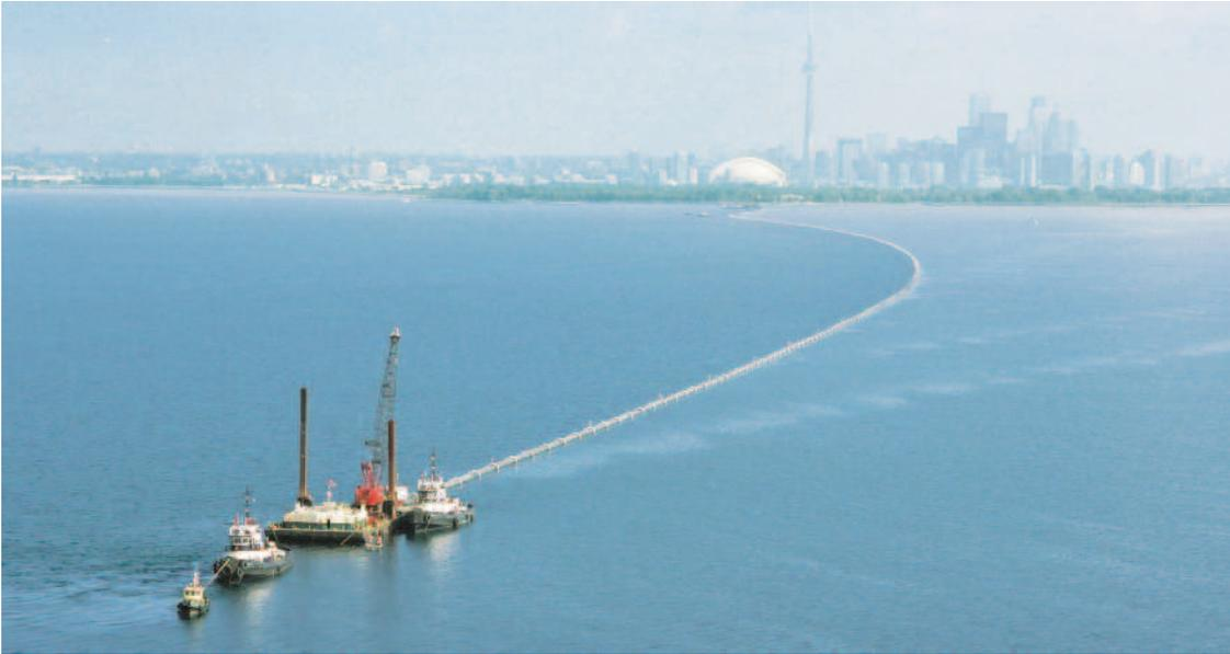
Thermal butt fusion provides an economical and fast method of delivering a complete, long, continuous length of pipe. Thermal fusion eliminates potential leak points every 8-20 feet commonly found with gasketed (or bell or spigot) pipe materials. The fused joints provide a continuous leak proof
