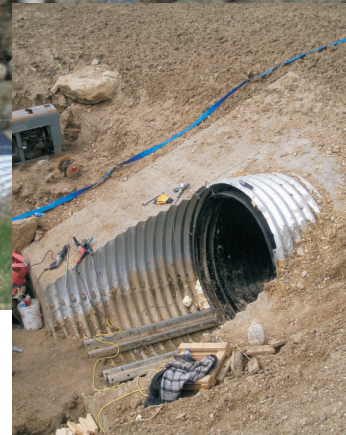
The last length of Weholite is successfully pushed into place.
