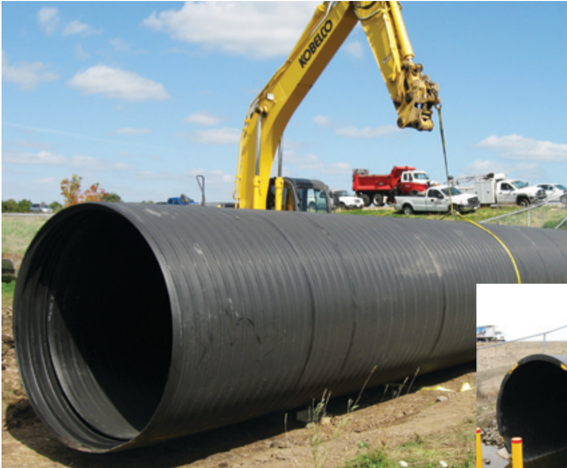
90"ID Weholite Liner is inserted into distressed CMP
