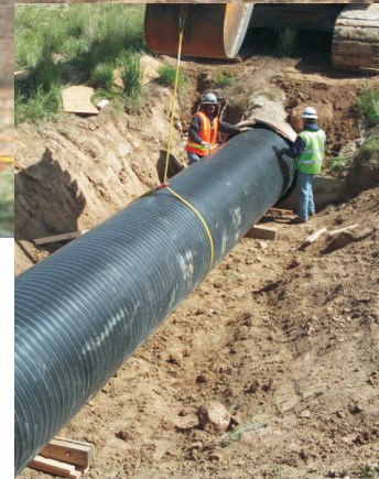
60' length of Weholite slips easily into existing culvert.
