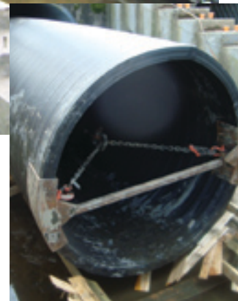
Weholite pipe being inserted into host pipe
