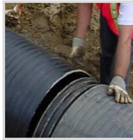
Step 2: Place pipes in straight alignment
