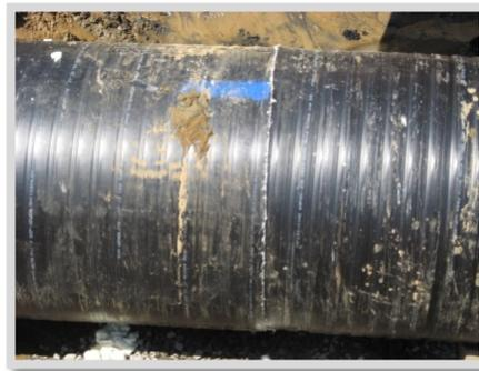
Step 4: Wipe off excess foam if necessary.
