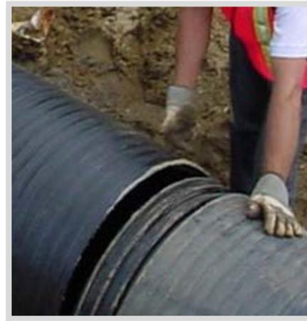
Step 2: Place pipes in straight alignment
