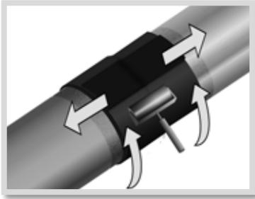
Step 16: While the sleeve is still hot and soft, use a hand roller to gently roll the sleeve surface and push any trapped air up and out of the sleeve, as shown above. If necessary, reheat to roll out air.
