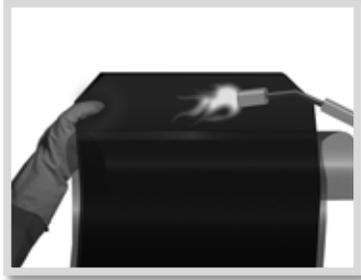
Step 7: Partially remove the release liner from the sleeve (~6" from the edge) and gently heat the adhesive along the underlap with a torch.
