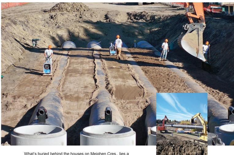
What's buried behind the houses on Meighen Cres., lies a sewer solution that is ready to work everyday for many years to come. Four parallel 1500mm diameter by 150 metre long Weholite tanks are connected to the sewer system and are located below the basements of the surrounding houses. The tanks collect sewage during heavy rainfall events and then gradual release it back to the sewer system where it can eventually be treated by the wastewater treatment plant.
