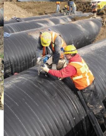
Uponor Technicians extrusion welding tank section
