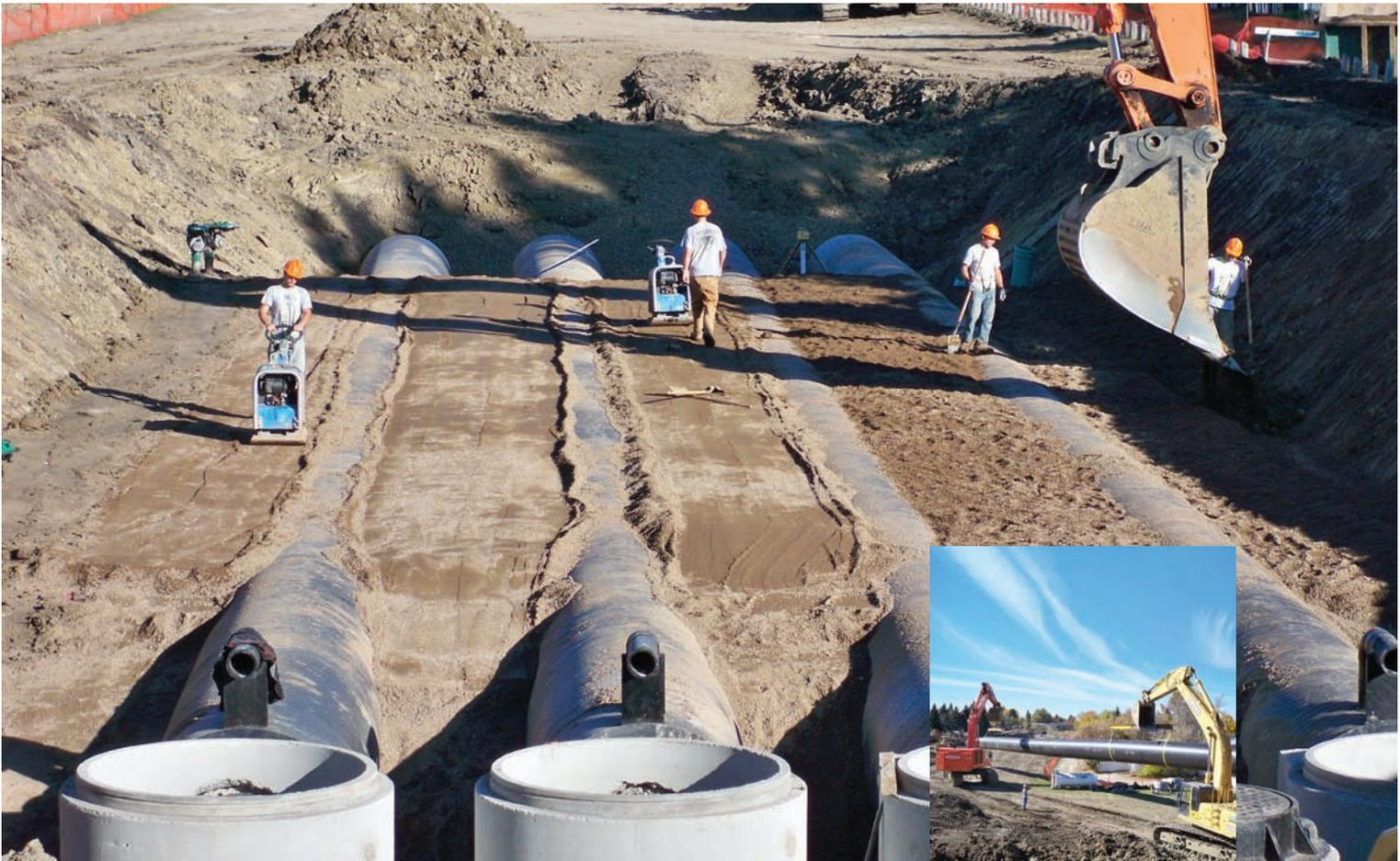
What's buried behind the houses on Meighen Cres., lies a sewer solution that is ready to work everyday for many years to come. Four parallel 1500mm diameter by 150 metre long Weholite tanks are connected to the sewer system and are located below the basements of the surrounding houses. The tanks collect sewage during heavy rainfall events and then gradual release it back to the sewer system where it can eventually be treated by the wastewater treatment plant.
