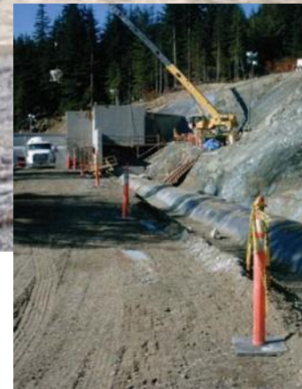
Remlayage - tuyau Weholite MD de 96 po
