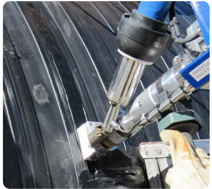
External Extrusion Welding
