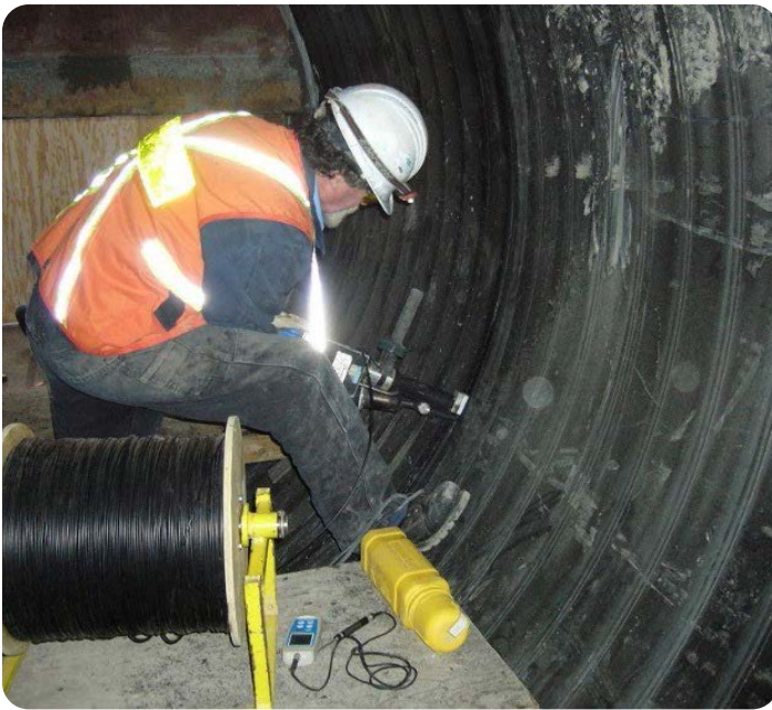
Internal Extrusion Welding
