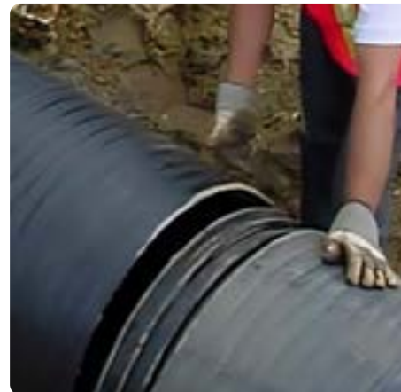
Step 2: Place pipes in straight alignment.
