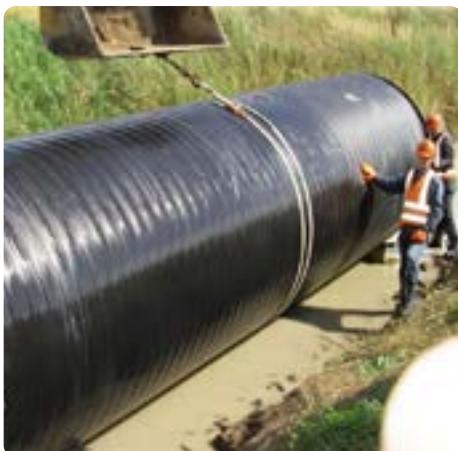
Step 3: Use nylon slings with a lever or excavator arm to rotate the pipe.
