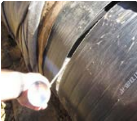
Step 1: Thread the pipe together until 1 complete turn is remaining to complete threading.
