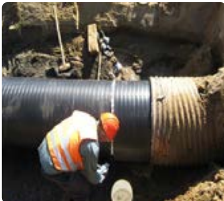
Step 3: Finish spinning the threaded joint until the thread no longer spins.
