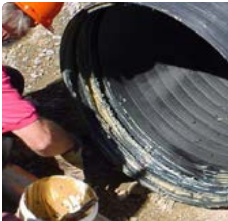
Step 1: Prior to threading the pipe, grease the threads to reduce the required threading force.
