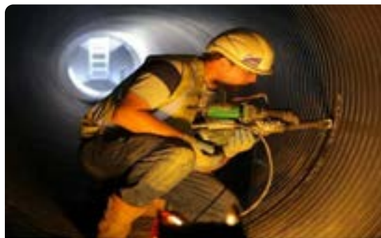
The inner wall weld
