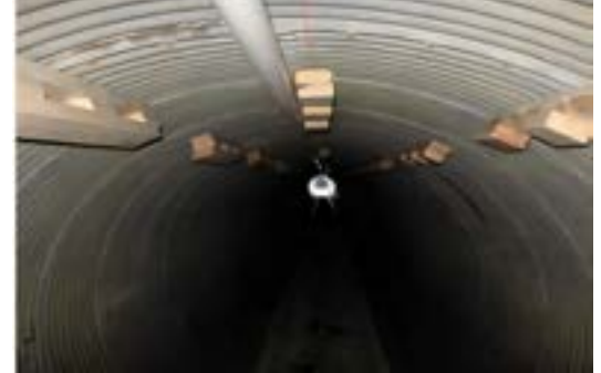
Wodden blocking at 10, 12, and 2 o'clock positions
