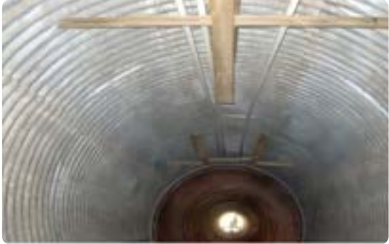
Wodden blocking that spans obvert of the pipe
