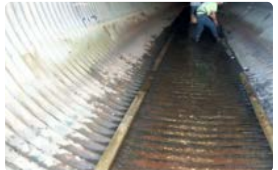
Wooden rails at the 5 and 7 o'clock position
