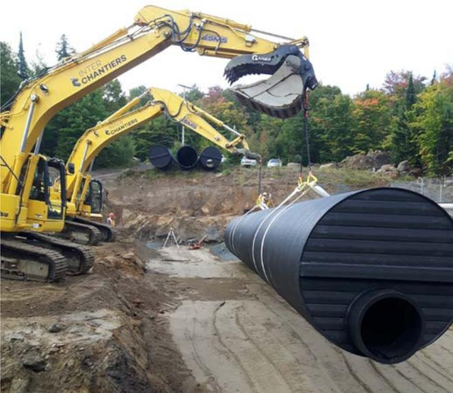
Infra Pipe's Weholite ASTM F894 profile wall structural polyethylene system provides a 100-year design life and is resistant to H<sub>2</sub>S, pH, corrosion, and abrasion. Weholite has been used throughout the world and North America since 1981.
