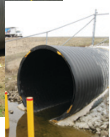
90"ID Weholite Liner is inserted into distressed CMP
