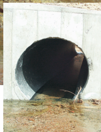
Weholite is easily adapted to accommodate a concrete head wall.
