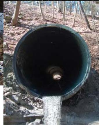
Weholite completely installed in the existing CMP culvert.
