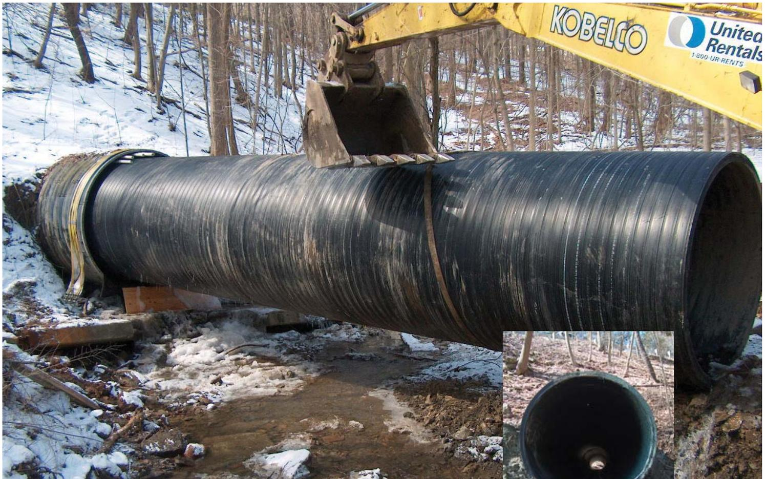
The residents of the village of Gates Mills, a quiet community just outside of Cleveland, were spared months of traffic and village disruption when Weholite was selected for their culvert rehabilitation project. The existing 120" CMP culvert was under 35' of cover and corroding badly.
