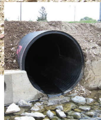
Sliplining 66" Weholite in pre-existing 84" CMP
