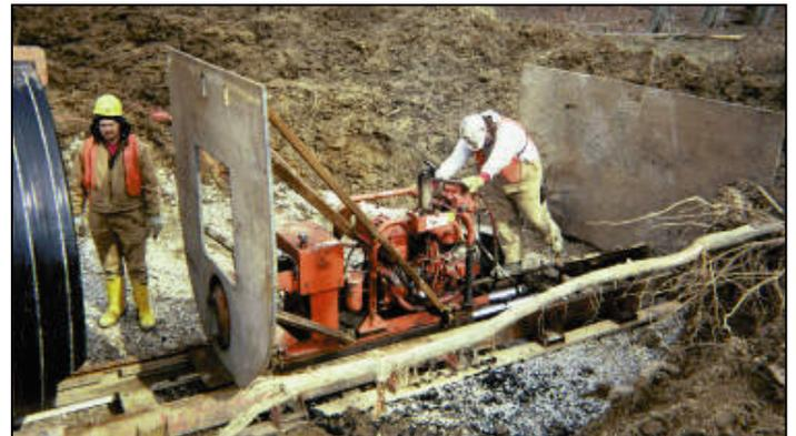
In Southern Indiana, a 96 inch corrugated steel culvert had become a threat to the major Interstate highway overhead. Premature corrosion had caused migration of the highway bedding into the culvert, resulting in a pavement settlement above.
