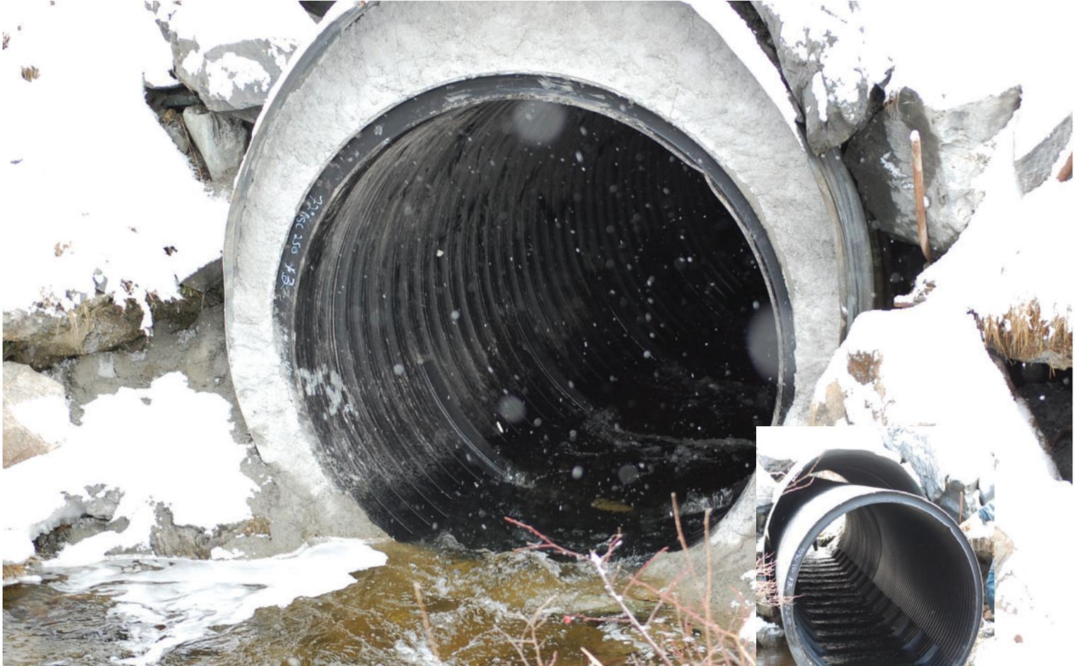
72" Weholite sliplined into existing CMP culvert
