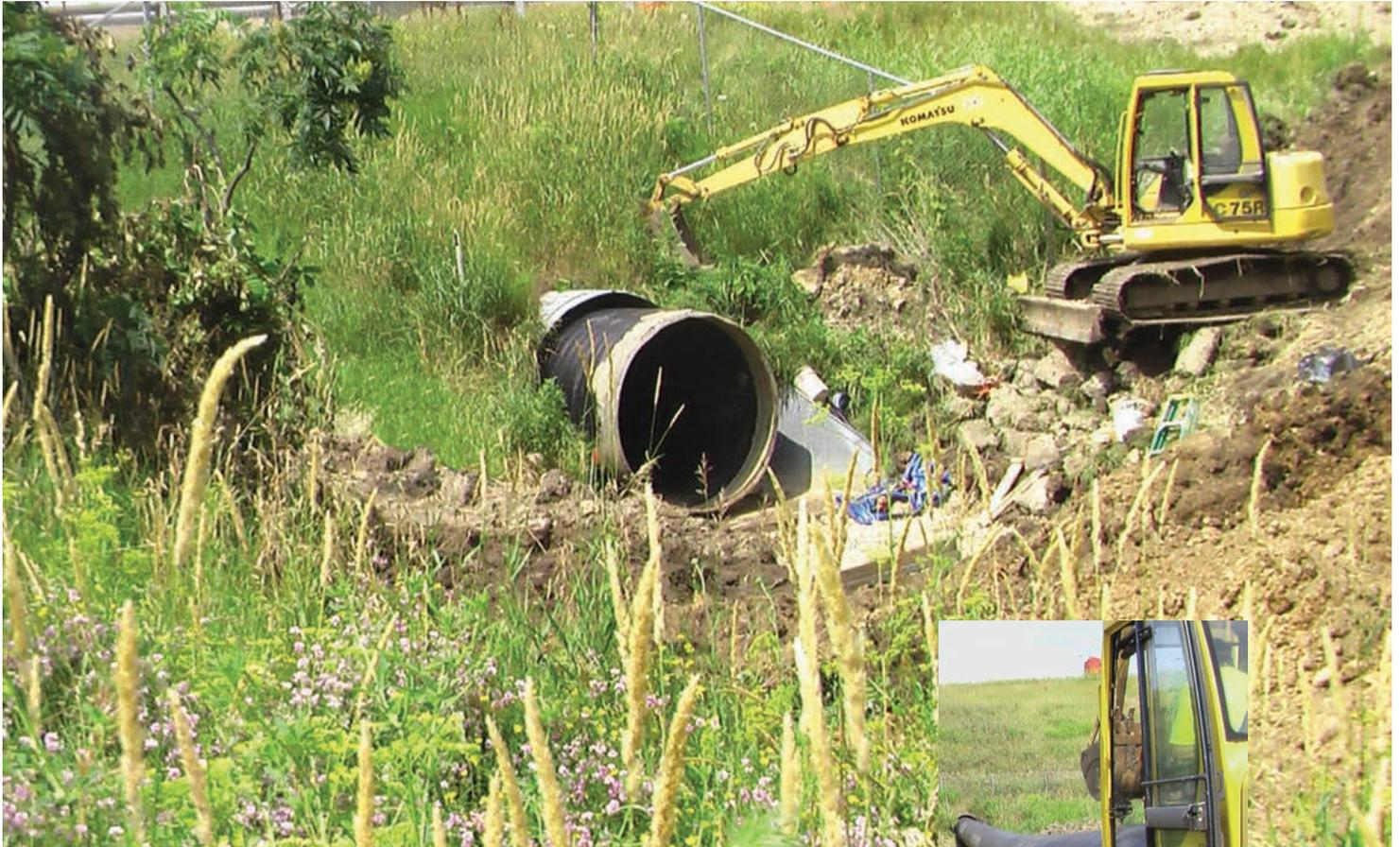
Early in 2008, the Wisconsin Department of Transportation (WI DOT) approved Weholite for culvert rehabilitation. The timing was significant as a major highway improvement project affecting the heavily traveled roads around Madison, Wisconsin was due to take place. Relining all existing metal culverts, approximately 50 in all, no matter the condition or extent of damage, was an integral part of this project.
