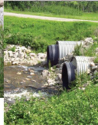
Weholite liners installed in two distressed metal culverts
