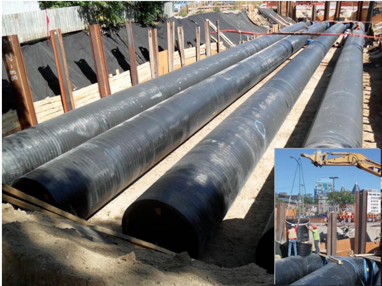
Placement of Weholite riser
