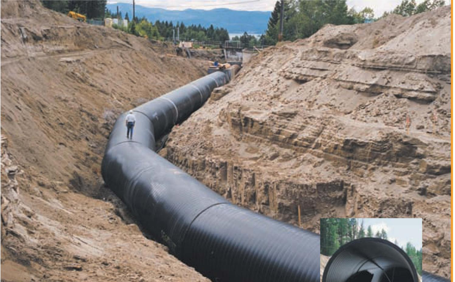
Pacificorp's Big Fork, Montana 4.1 MW hydroelectric power plant has been in service for over 100 years. Weholite was selected to replace a woodstave penstock feed line that parallels the Swan River. After many years of service, in 2000, a failure of the woodstave pipeline caused a washout into the scenic Swan River, along a section of the river that is popular for canoeing and whitewater rafting. The plant's electrical output was cut in half, pending replacement of the pipeline.
