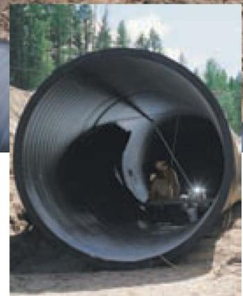
Full wall welds using an automated extrusion welder.
