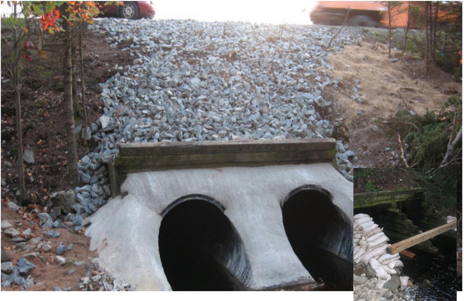
NST&IR selects a trenchless construction method to rehabilitate a failing timber box culvert under one of Nova Scotia's busiest highways. The project located along Hwy 102 required the contractor to slipline a 1.83m high, 3.66m wide and 38m long timber box culvert with two 125' by 54" RSC250 Weholite pipes.
