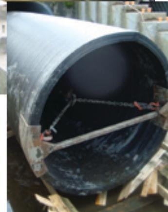
Weholite pipe being inserted into host pipe
