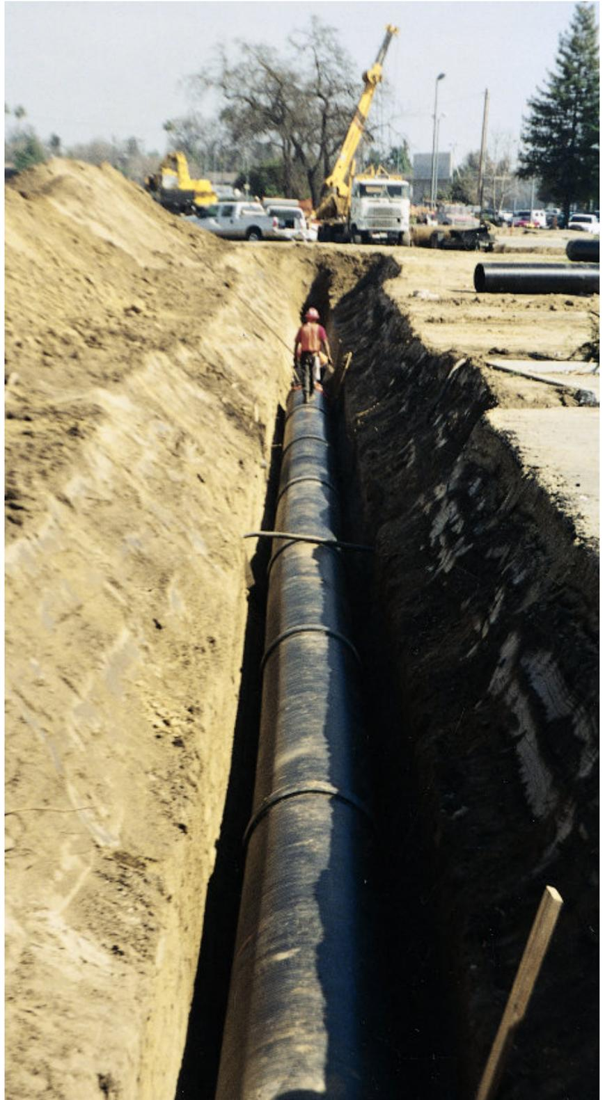
In March of 1999, Rising Sun Construction, Inc. began construction of a major bypass improvement sewer on state highway 198 located in Visalia, California. Included in the scope of the project was the installation of 7,300 linear feet of 30" diameter Weholite to be used as an outfall line. This sanitary sewer line was subsequently turned over to the City of Visalia after completion of the project.
