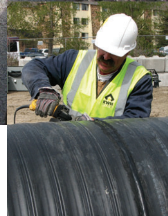
Uponor's technician prepares the pipe
