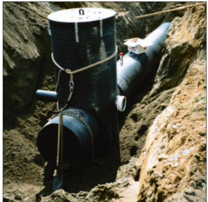
remediation costs, use native material for backfill and maintain the same flow as 36" concrete pipe while maximizing ground cover. Based on the significant savings in material and installation, the district is now considering using HDPE pipe in an increasing number
