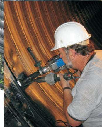
KWH Pipe field welding technician performs an extrusion weld on 120” ID Weholite tank.
