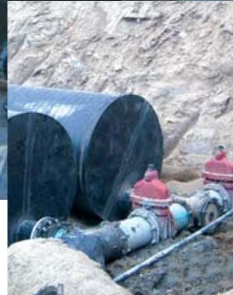
Inlet/Outlet Valve Train for Chlorine Contact Pipe.
